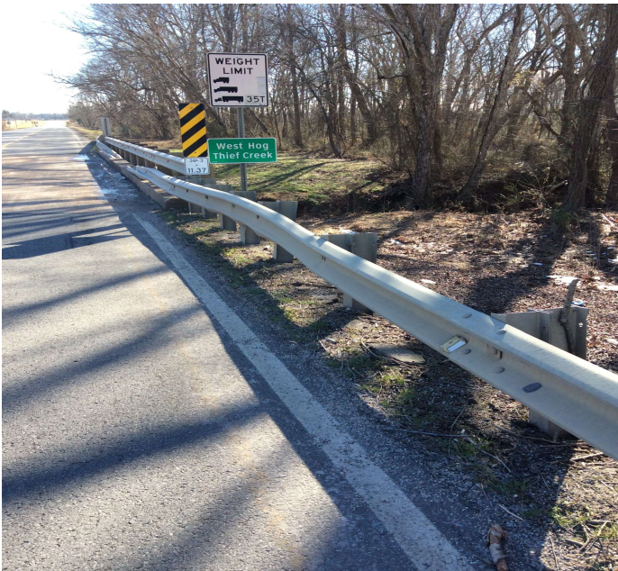
PHOTO 1 Description 14' guard rail bent on Right at approach at Abutment 1.
