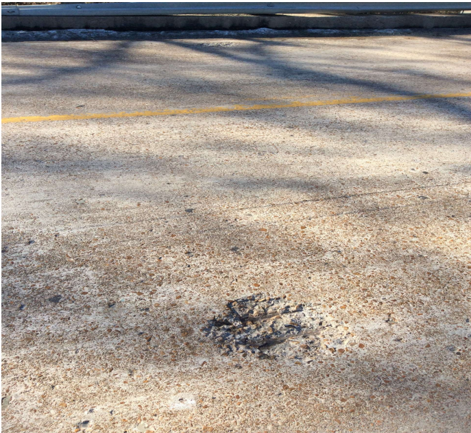
PHOTO 1 Description Spalls to deck with rebar exposed @ Span 1 & 2.
