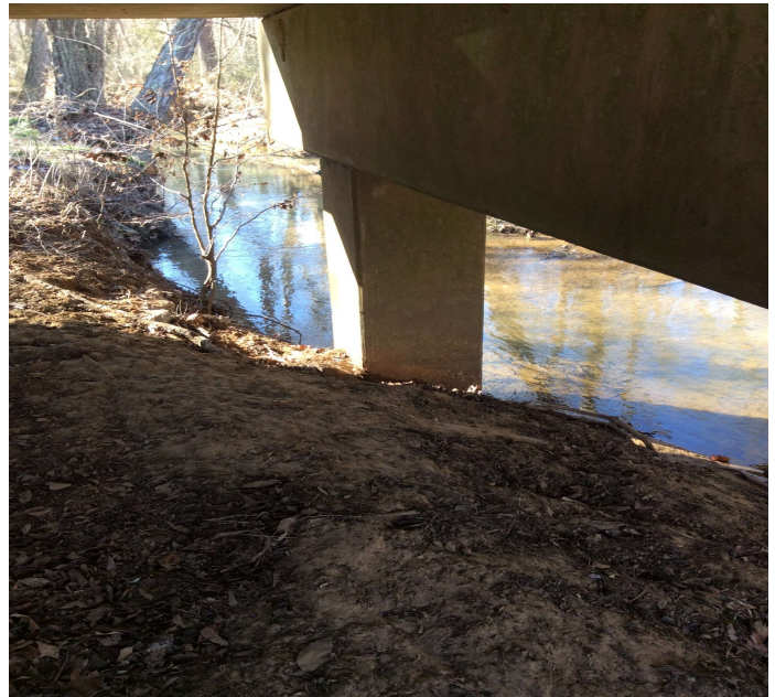
PHOTO 2 Description Scour to Right column at Bent 2.
