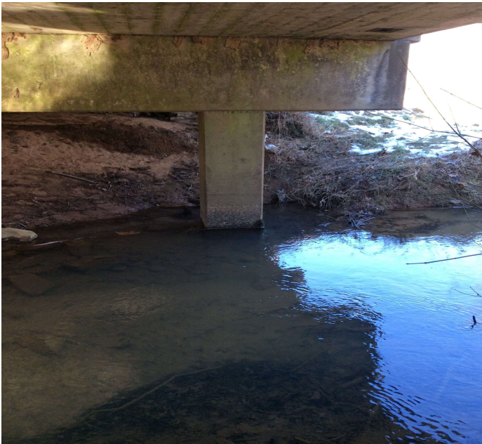
PHOTO 1 Description Scour to Left column at Bent 1.
